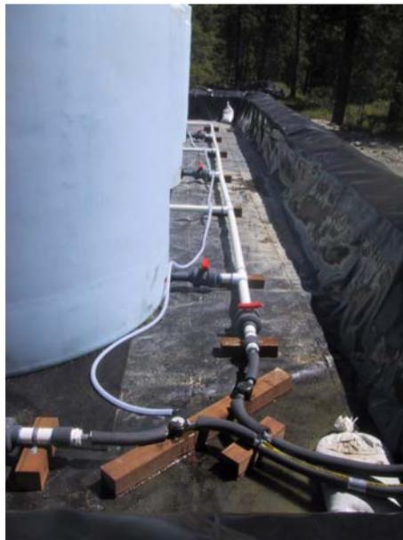
**Figure 6. Outflow Arrangements for Nutrients, Showing Small In-line Filters**
