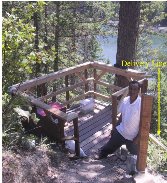
Figure 8. Platform for Control Box, Showing Delivery Line (bottom left)
