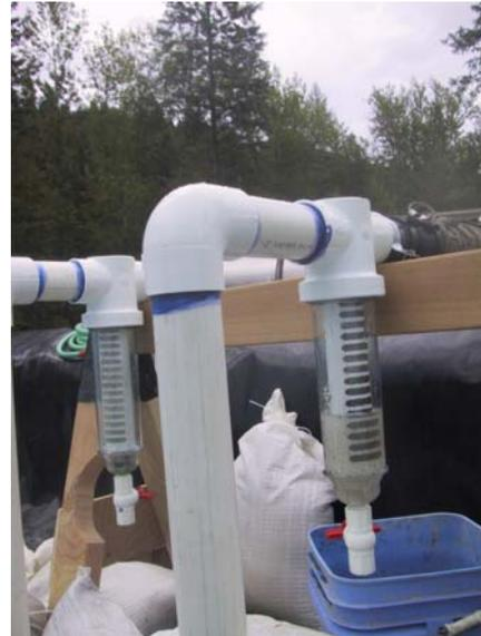
**Figure 3. Filling Arrangements for Tanks Showing Connectors and Filters.**
