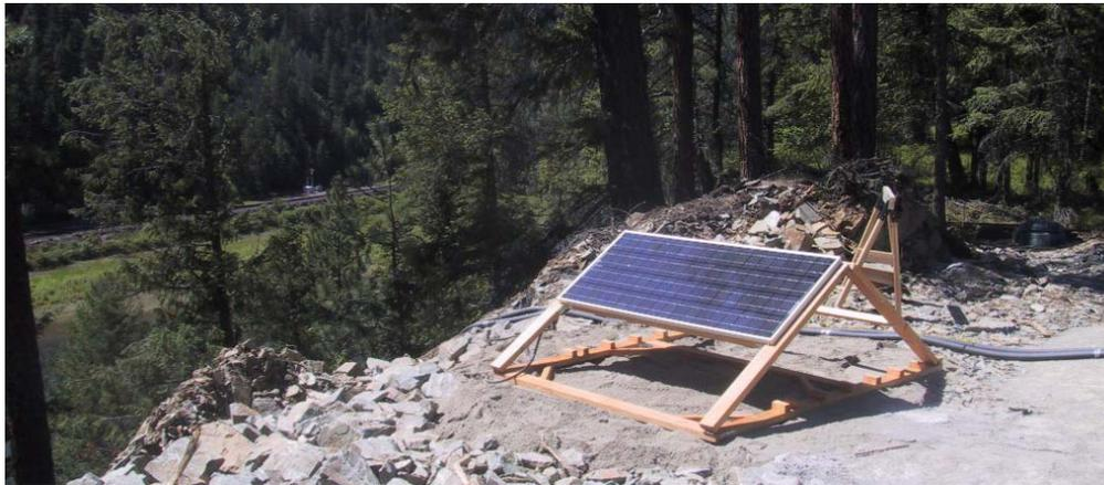
**Figure 12. Photovoltaic Panel, Showing Adjustable Mount for Sun Angle**
