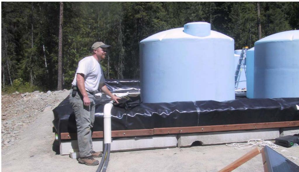
**Figure 2. Tanks for Storing Liquid Nutrient
